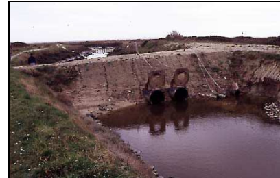
Earthen dam with flap gates
