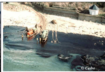
Pumping oil at the bottom end of the foreshore – the Tanio spill
