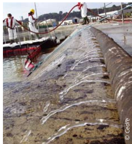
Water curtain to protect a quay or slipway.
