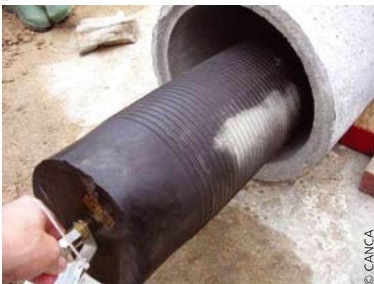
Introducing an inflatable stopper into a waste water evacuation pipe.
